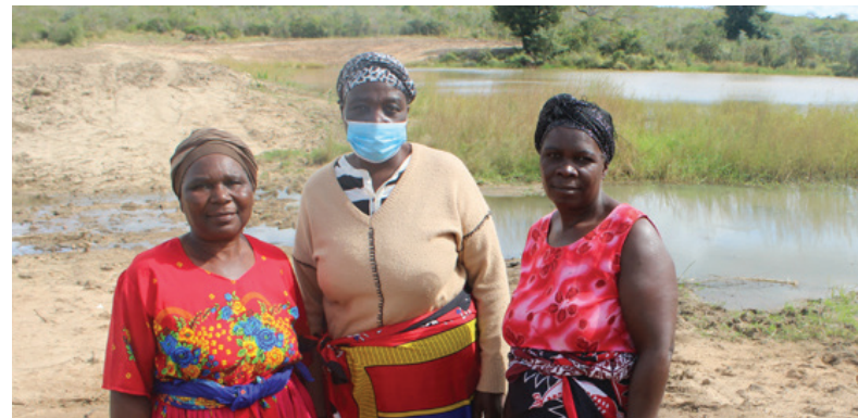
Mrs Margaret Mnisi, Suzanne Silauhe and Annya Mkontso at the collapsed dam wall in Ireagh Village in the Bushbuck Ridge area.
